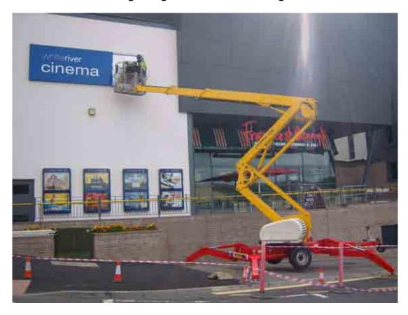
The **Nifty 210** has one of the largest unrestricted working envelopes in its class. Hydraulic outriggers make it quick and easy to set up and an optional traction drive system, operated from the platform, allows the 210 to be positioned on site with minimal effort. Platform rotation provides greater manoeuvrability in the air and its fully proportional controls give the operator precise control when positioning the platform, even on hard to reach jobs.
